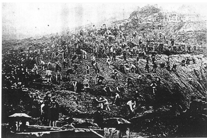
Fences being torn down on Plumstead Common, 1876
